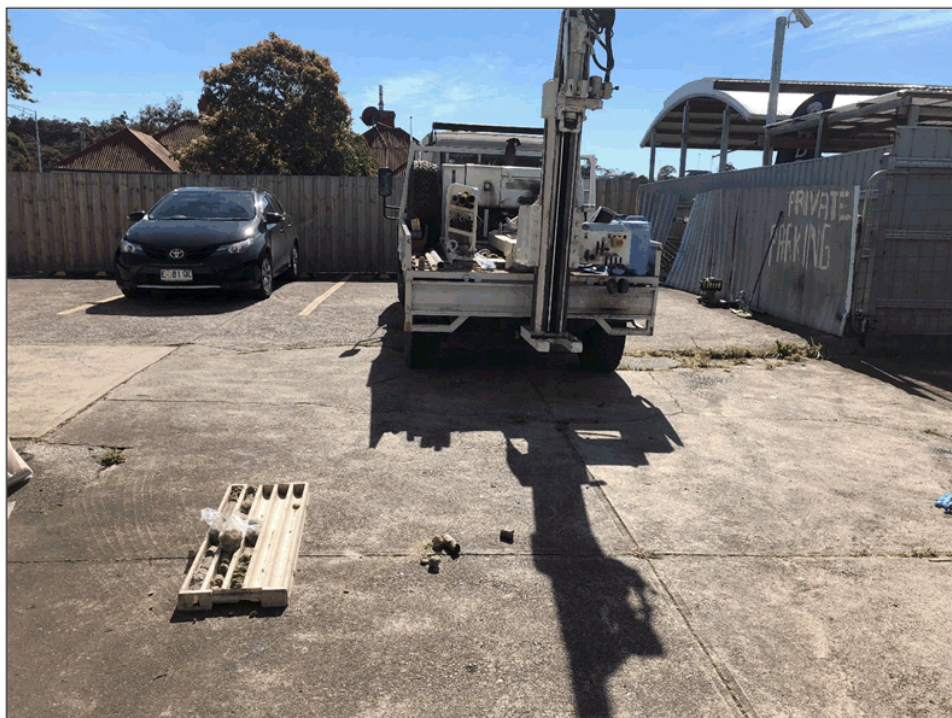
Plate 3 One of the Investigation Holes Drilled Near the Underground Storage Tank
