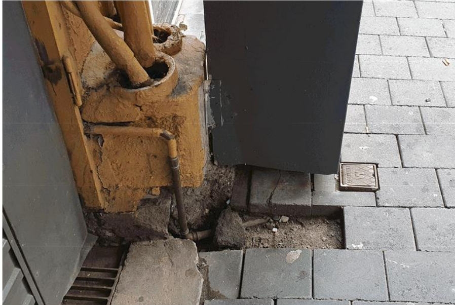
DN25 domestic water connection at rear of building.
