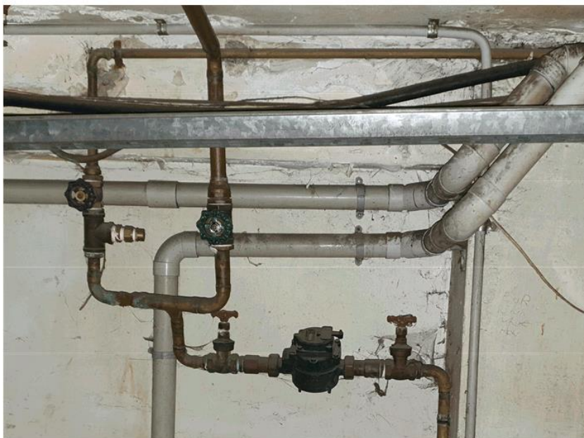
DN25 water meter located in basement.
