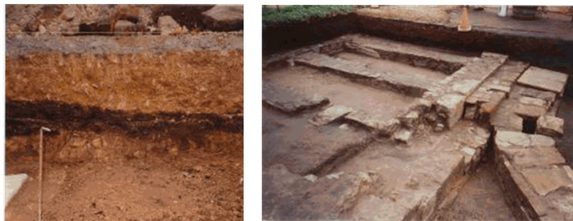
Figure 19 Views showing depth of overburden/fill and resulting solitary apartment footings from test excavations in Yard 3.
