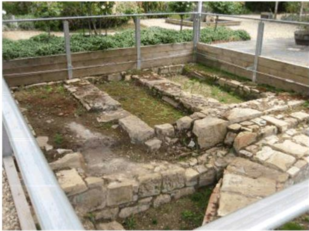
Figure 30 This image shows the same view today. Note vegetation encroachment and mortar deterioration both due to excessive rainwater.
