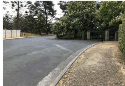
16. Existing path requires resurfacing to enable shared use.
