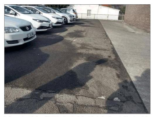
Surface covering at the front of 48-50 New Town Road, view to the South, red concrete slab under asphalt
