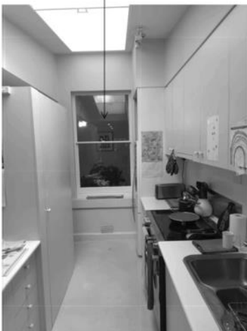
existing window between dining room & kitchen to be removed (photo from kitchen looking towards dining room)
