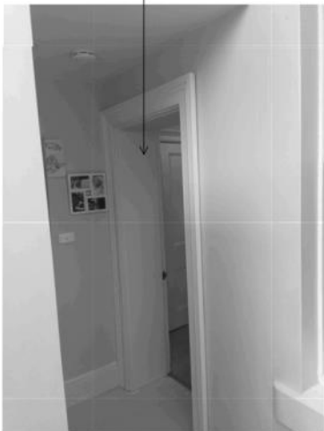
existing door between dining room & kitchen to be removed (photo from kitchen looking towards dining room)
