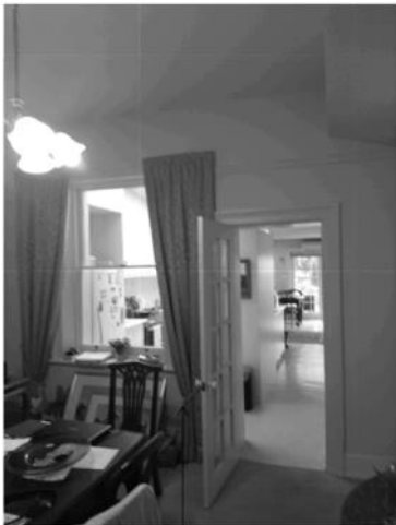
existing wall between dining room & kitchen to be partly removed to a height of 2375 mm (photo from dining room looking towards kitchen)
