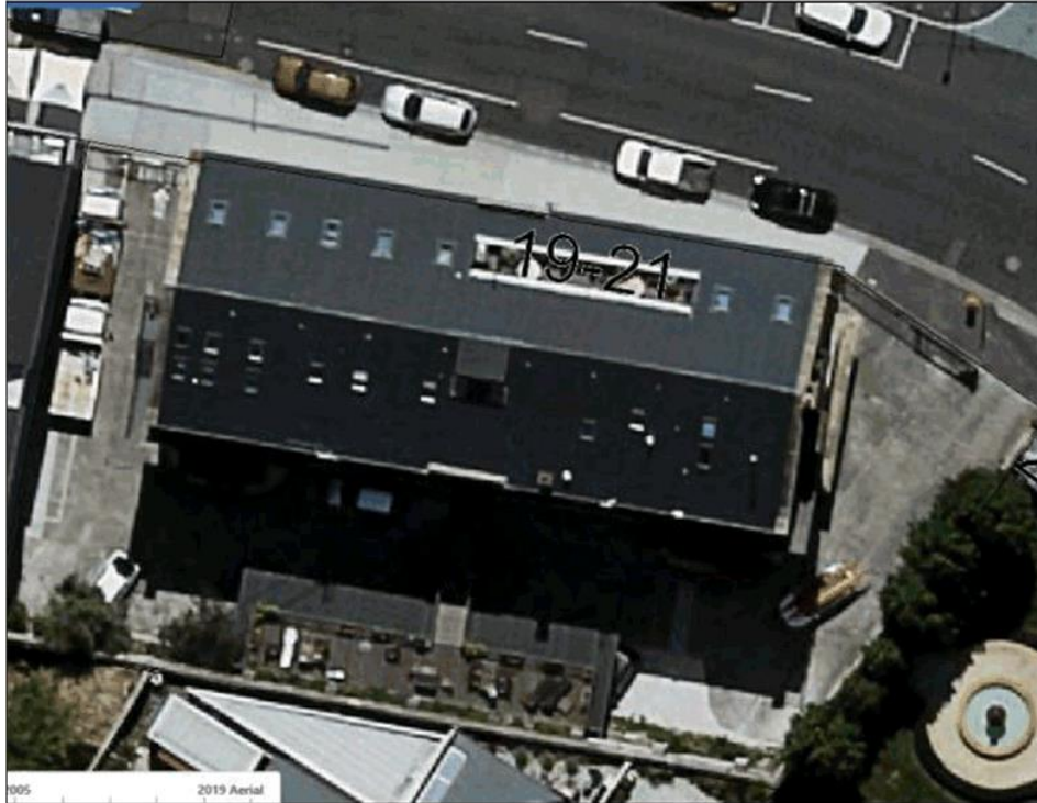
Figure 2 above: aerial photograph of subject site and Castray Esplanade frontage.
