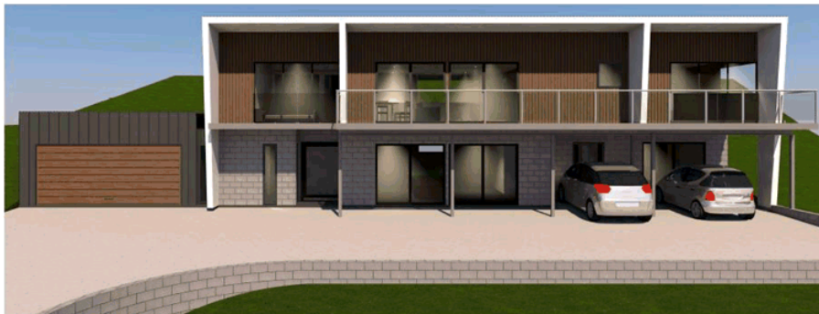
Figure 5. The building design of the east (front) showing the extent of the pergolas and eaves over glazed areas (from Modern Architecture Practice, ref: BA01)
