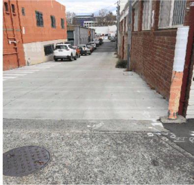
Existing stormwater pit for possible new connection (in foreground) – looking down laneway towards the existing connection in the background (behind the tuft of grass)
