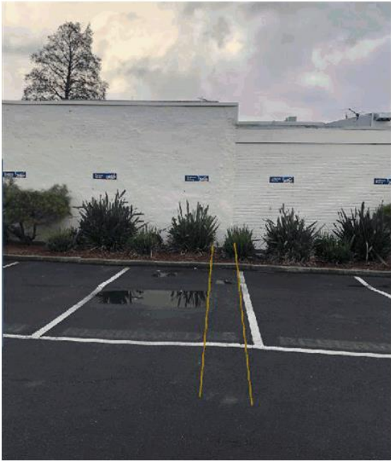
Figure 6.4 – Example of pavement cracking in-line with expected rear wall of the c1890s building.
