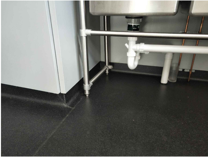
EX. FLOOR FINISH & COVING PREVIOUSLY COUNCIL APPROVED AS AS 4674 COMPLIANT. EXISTING COVERED SHEET VINYL SKIRTING = 100mm HIGH. EXISTING FLOOR FINISH SLIP RATING PREVIOUSLY APPROVED.
