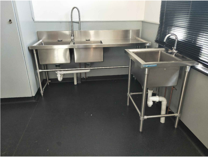
EX. WASH & FOOD PREP SINKS PREVIOUSLY COUNCIL APPROVED AS AS 4674 COMPLIANT
