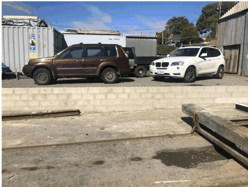
Figure 4.3 – Modern fill and retaining wall benching the shoreward portion of the western part of the site.
