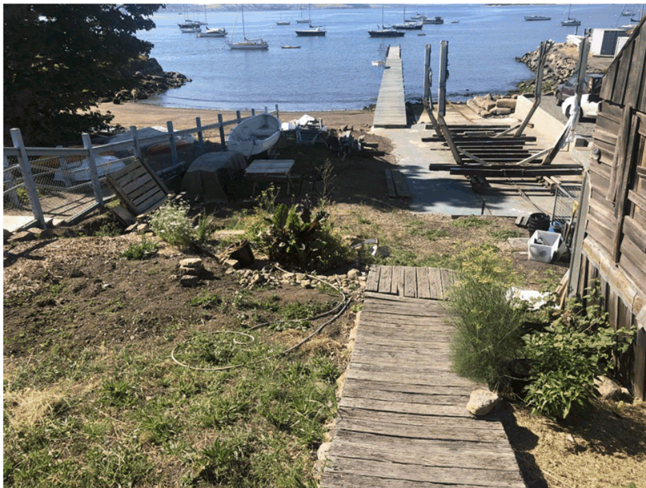
Figure 4.1 – View across the slip site from the top of the site.
