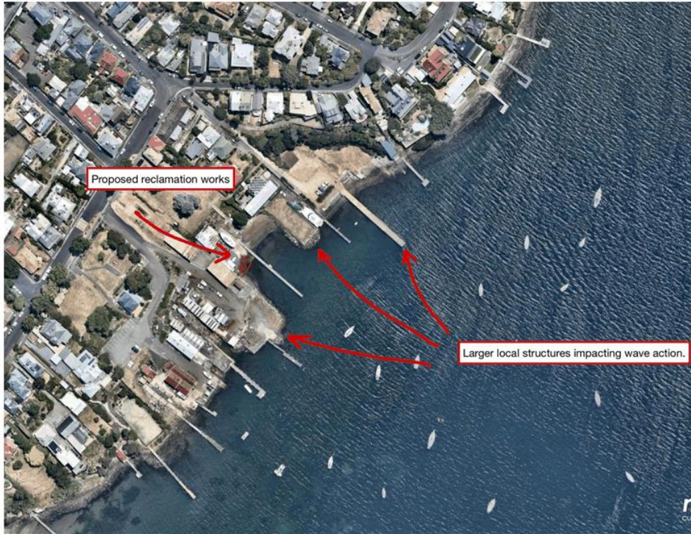
Figure 2: Wide view image showing wave action impacted by larger structures but not by modest size of proposed reclamation works
