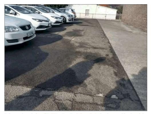
Surface covering at the front of 48-50 New Town Road, view to the South, red concrete slab under asphalt
