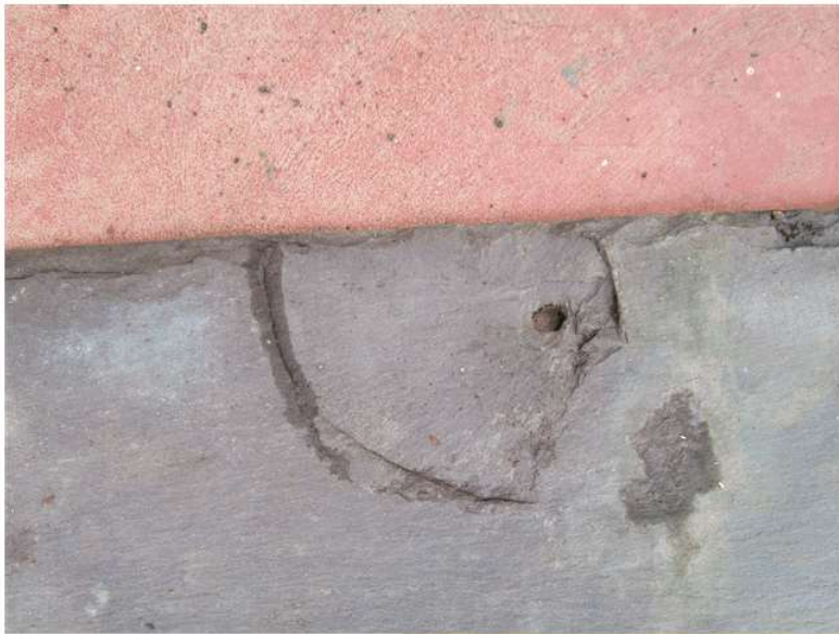
Fig 1: Eroding edges of roof slate
