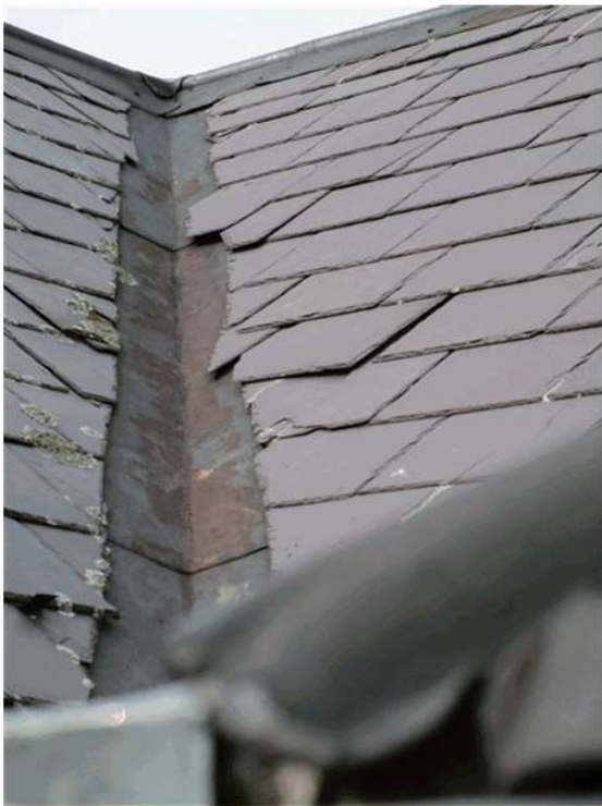
Fig 2: Rusting valley flashings and loose slates
