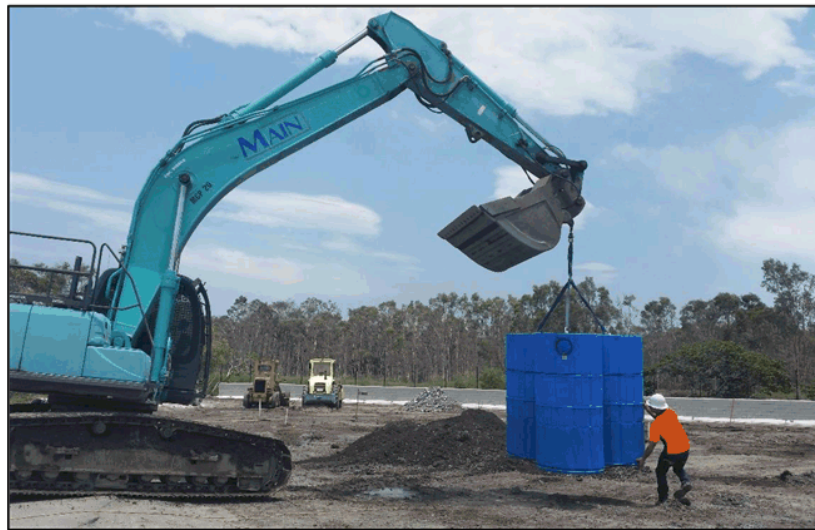
Figure 4.3: SPEL Hydrosystem (SHS.1000) installation using onsite digger
