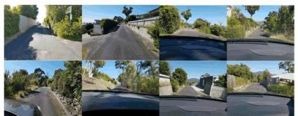
Figure 11 (Image 5 of Senior Development Engineer's Report): Sight distances along Niree Lane from driver's perspective (note car is a 4wd with slightly elevated seat height)
