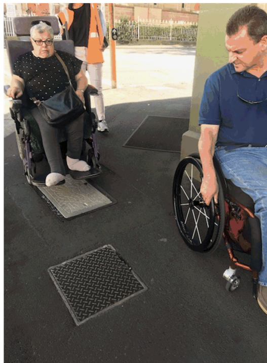
Inspecting the footpath surface. If pit lids are not maintained they can become hazards for wheels and heels alike.
