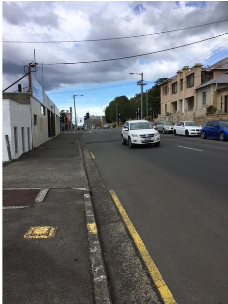
Photograph 10: Showing sight distance along Harrington Street exceeding the 80 metre requirement for a 50km/hr road.
