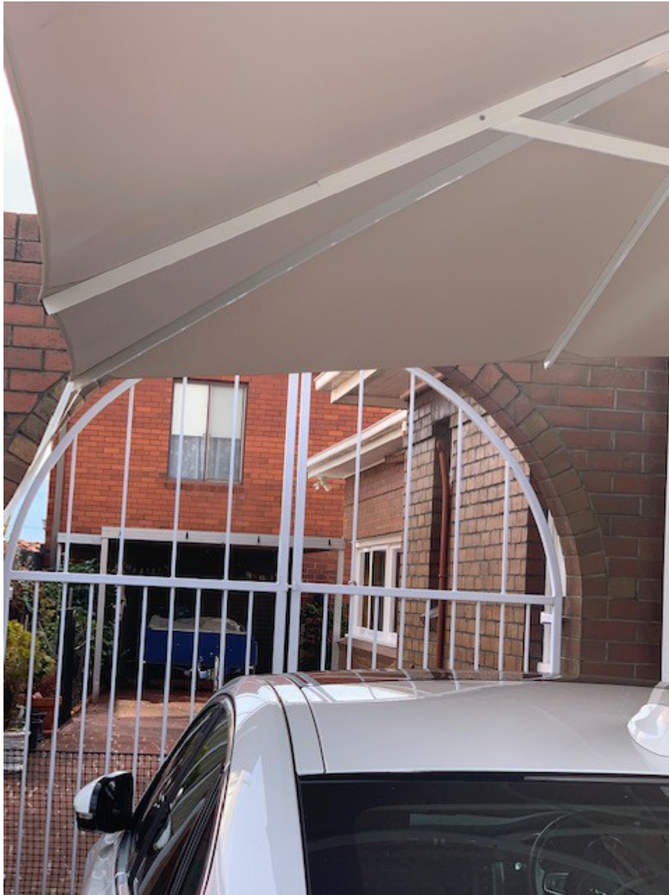
Figure 3: Existing garage and carport (officer photo, 2019)
