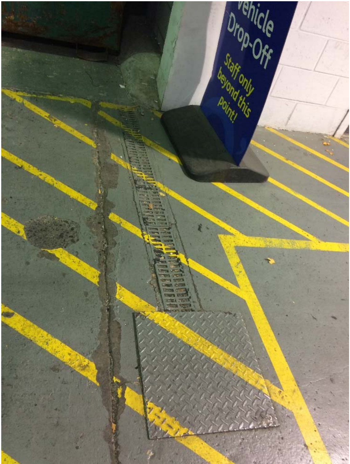
Plate 2 Partial grate across one side of vehicle access way, adjacent washdown area
