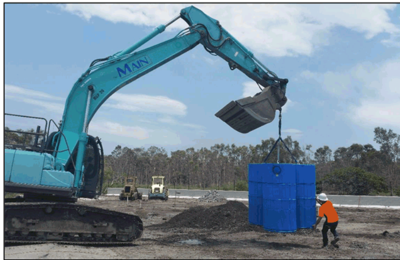
Figure 4.3: SPEL Hydrosystem (SHS.1000) installation using onsite digger
