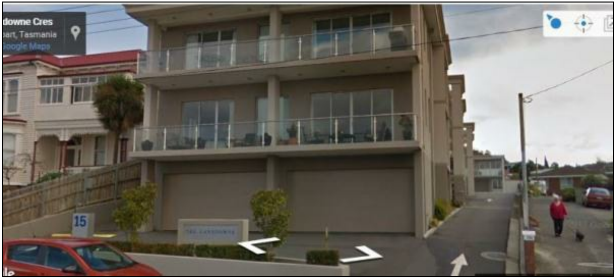
Figure 3: image of facade. Source: Google Streetview.
