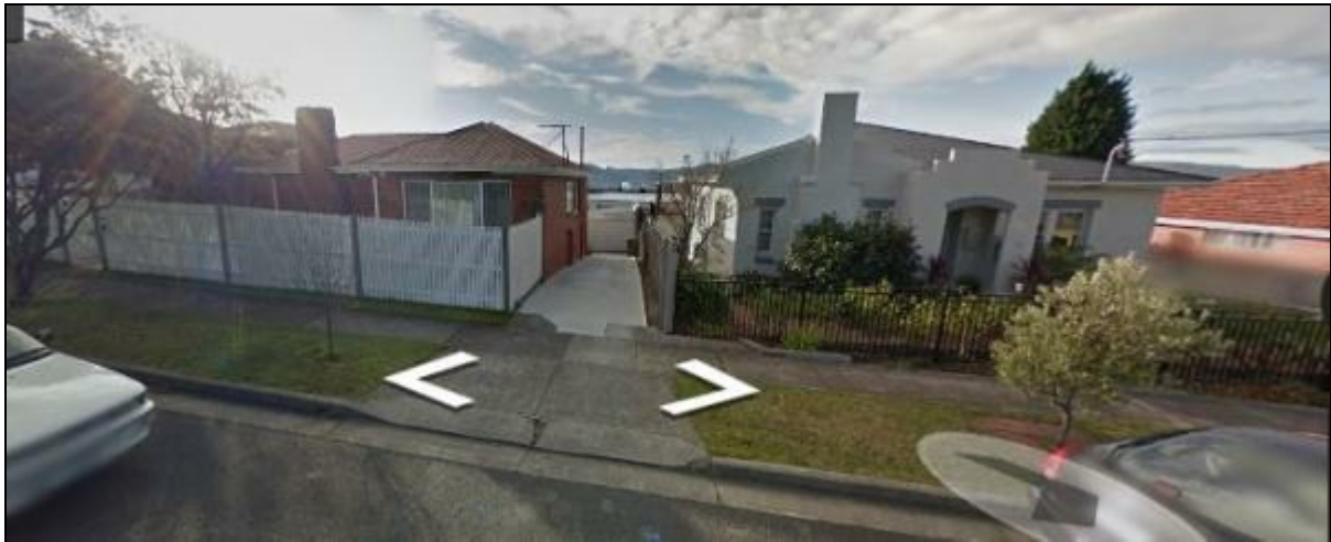
Figure 3: Google Streetview showing the applicant site to the right, and No.5 Raymont Terrace (including driveway and rear garage) to the left.
