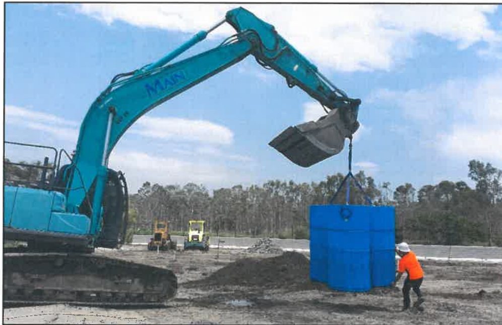
Figure 4.3: SPEL Hydrosystem (SHS.1000) installation using onsite digger
