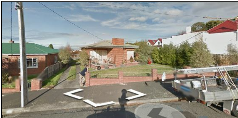
Figure 3: 52 Hamilton Street, from Google Streetview.
