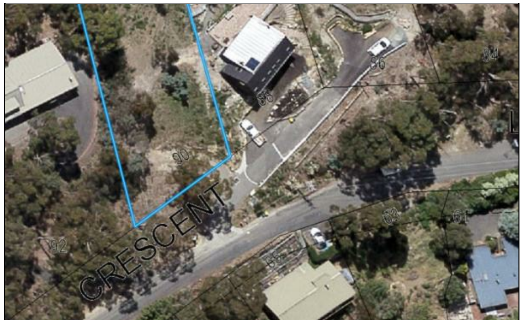
Fig. 7. View of part of the subject property.
