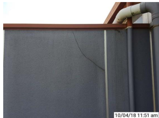
External Wall Cracking
