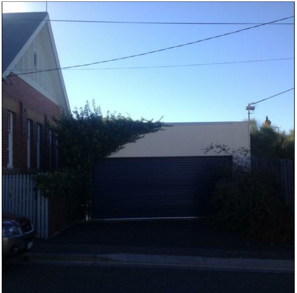
Figure 16: Existing garage adjoining 51 Feltham Street.
