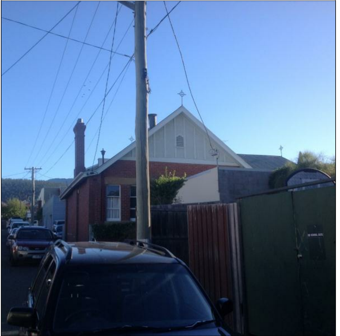
Figure 5: Looking north west towards site and the existing red brick building of 51 Feltham Street.
