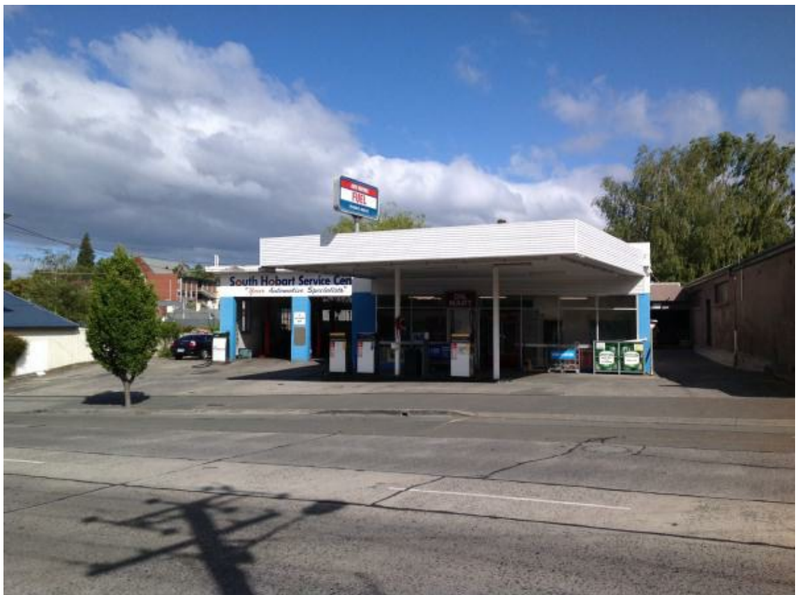
Figure 3: Site as existing with service station and service centre to be demolished
