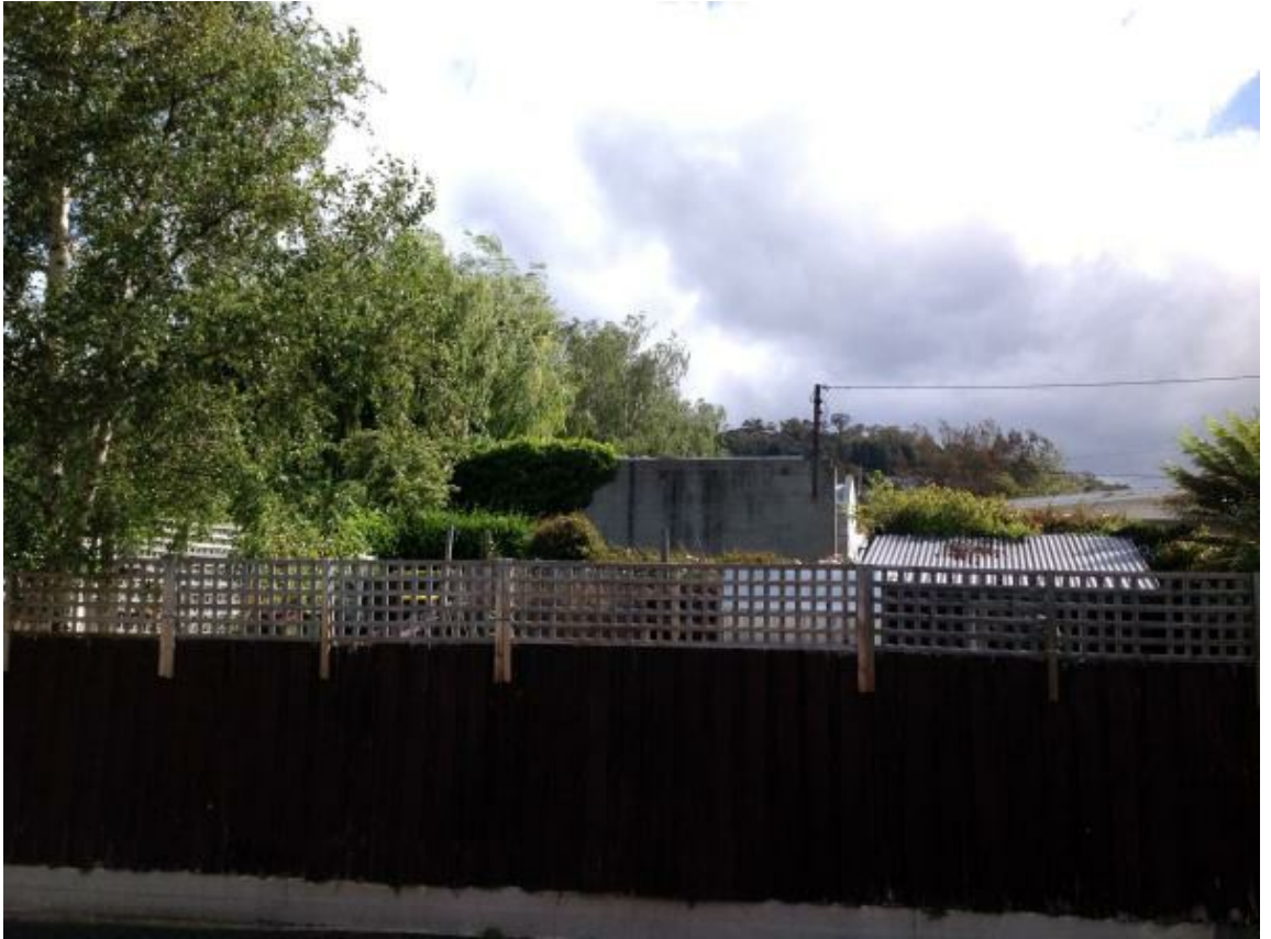
Figure 5: Wall of existing motor vehicle repair workshop as viewed from Denison Street.
