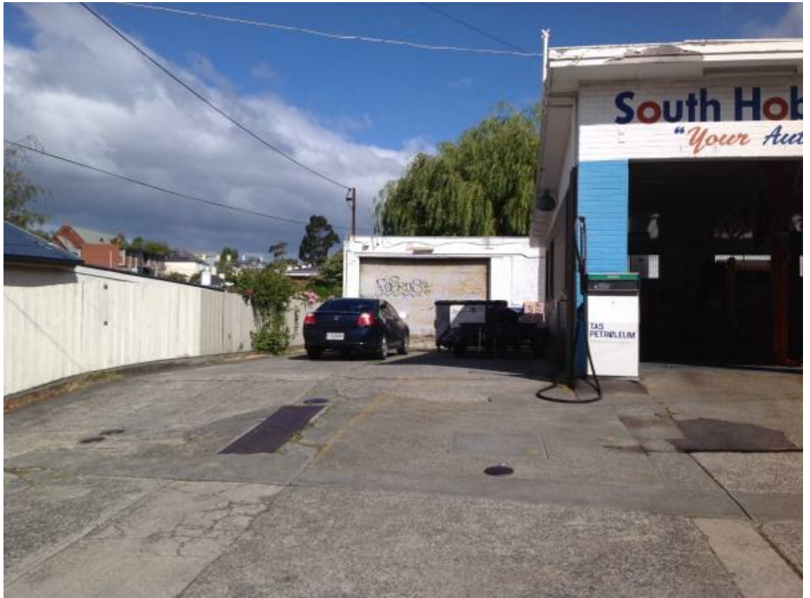
Figure 4: The motor vehicle repair workshop to the side of the service station and service centre is proposed to be extended, have its walls replaced to the same height as existing and have a new gable roof.
