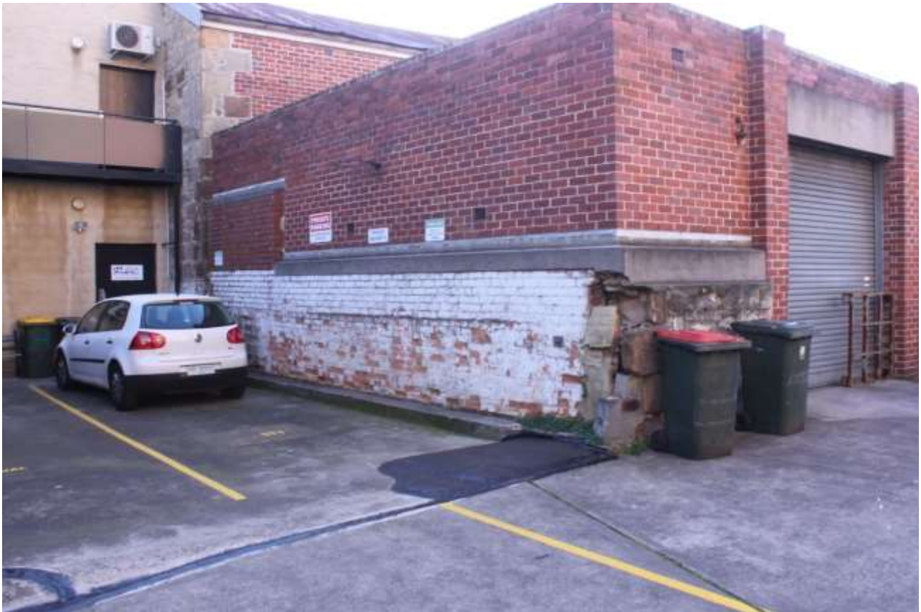
Figure 3.5.1 – The 1964 rear extension of 25 Salamanca Place, showing earlier fabric incorporated, probably from earlier development at 23 Salamanca Place.
