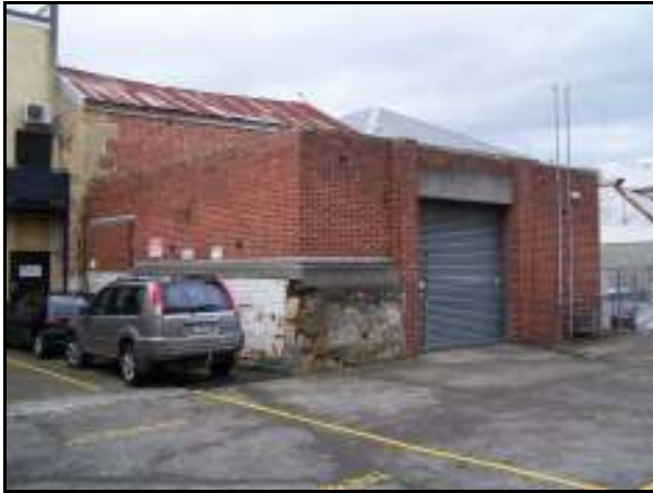
Figure 4 Note the earlier brick and stone foundation
