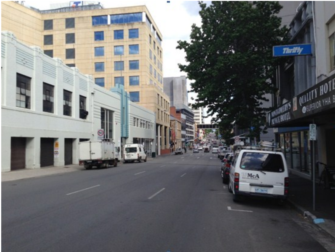
Figure 3: Existing view up Argyle Street from near Macquarie Street intersection.
