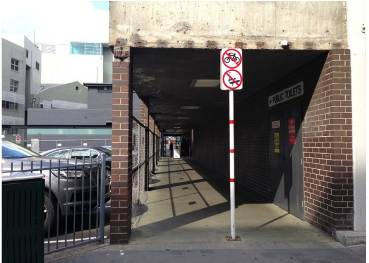
Figure 6: The existing Argyle Street car park walkway which would be demolished and replaced by the retail arcade which would be located to the left of this picture.
