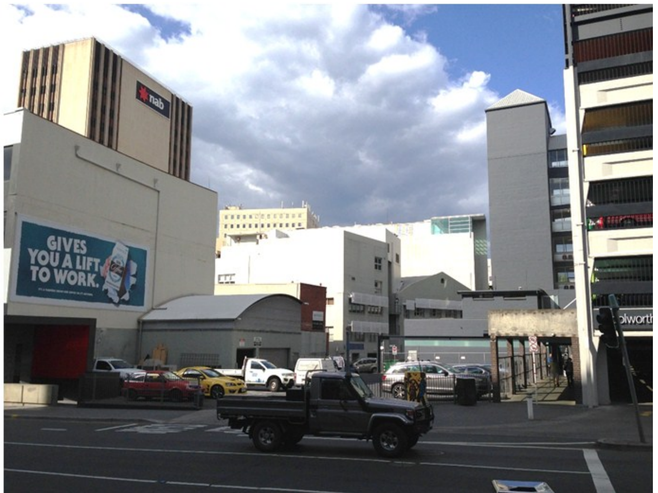
Figure 5: The site of the proposal from the opposite side of Argyle Street. The curved roof structure is the garage/shed building which is to be demolished.
