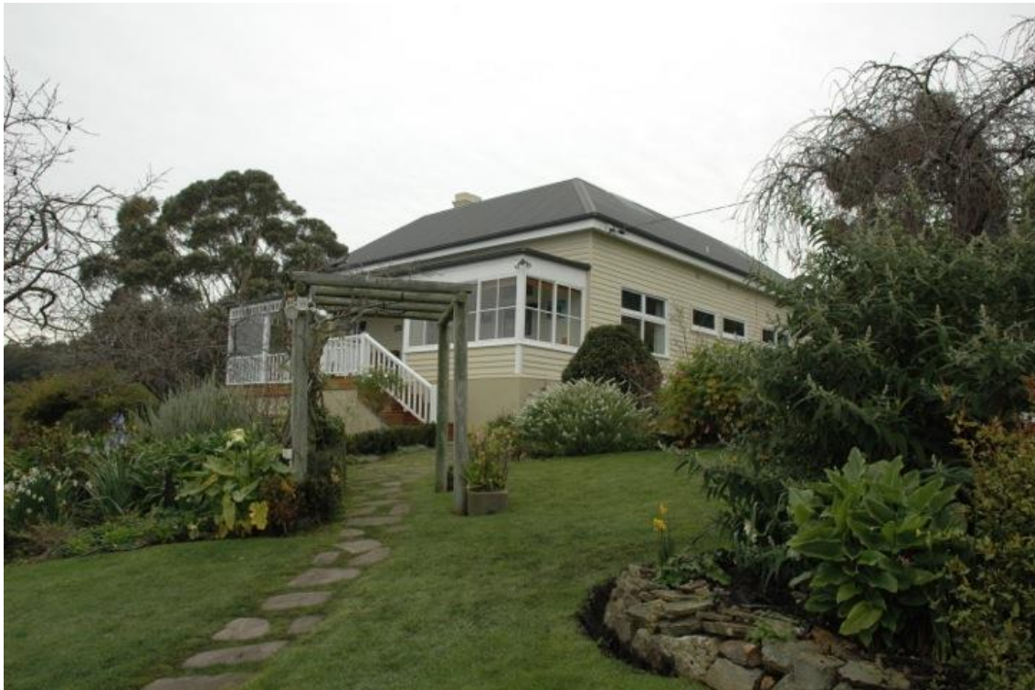
Photo 4: The heritage listed house at 1 Folder Street.
