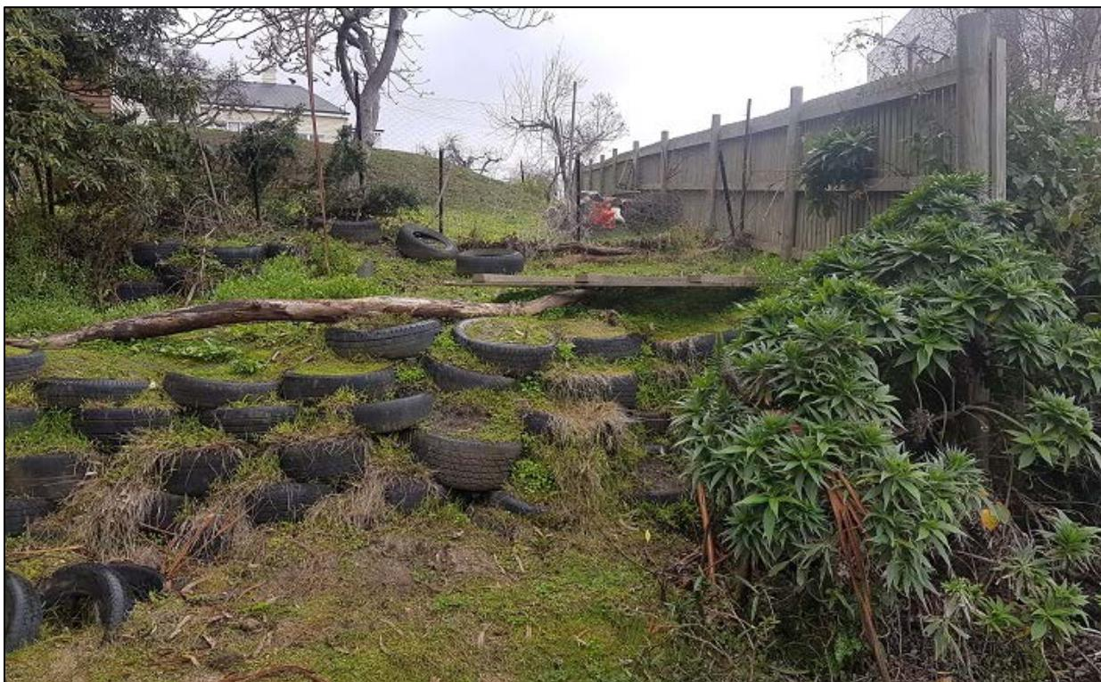
Figure 3 – Bank retained with old car types at boundary of land to be transferred to HCC.
