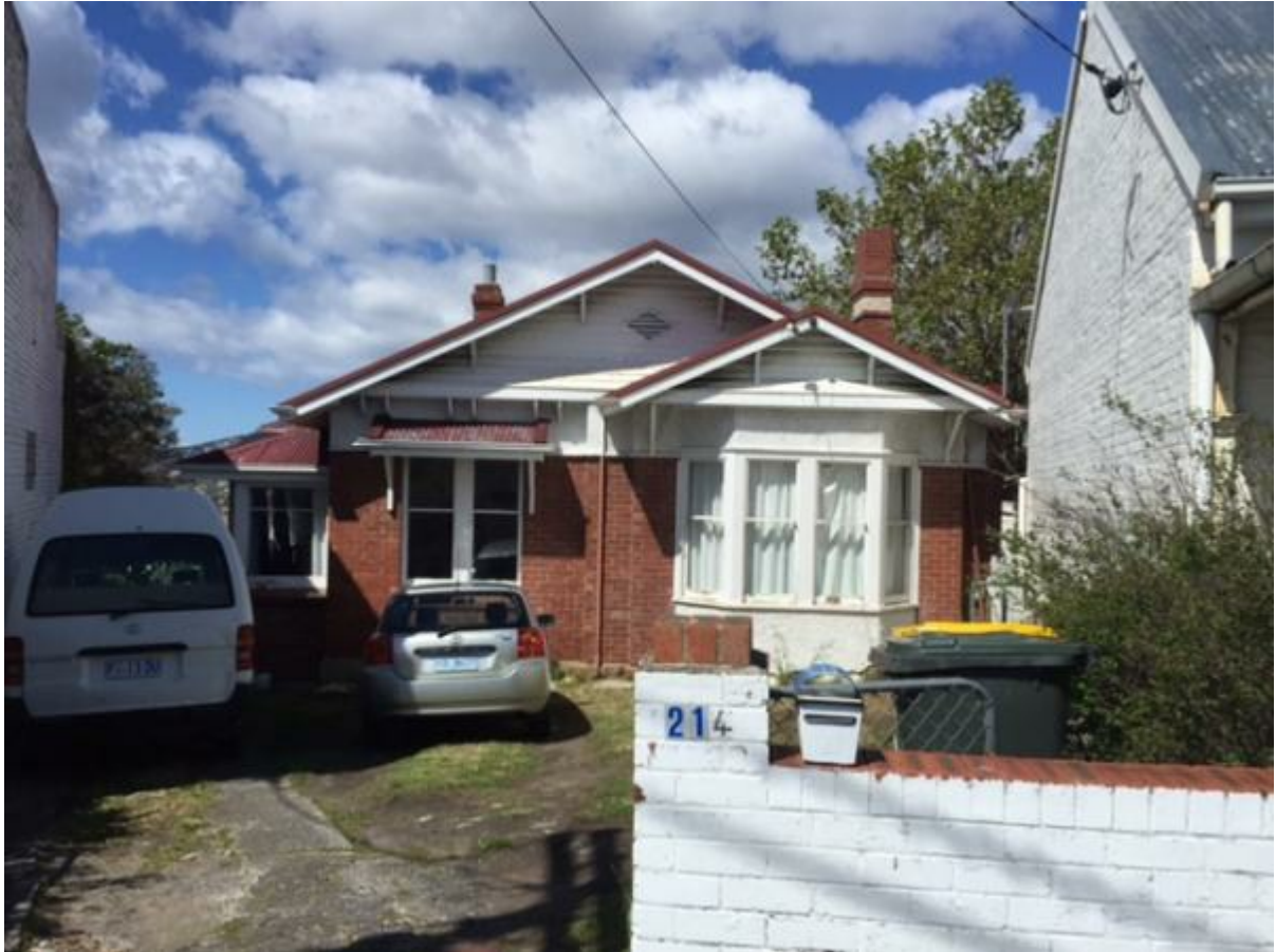
Figure 2: The property as viewed from Melville Street.
