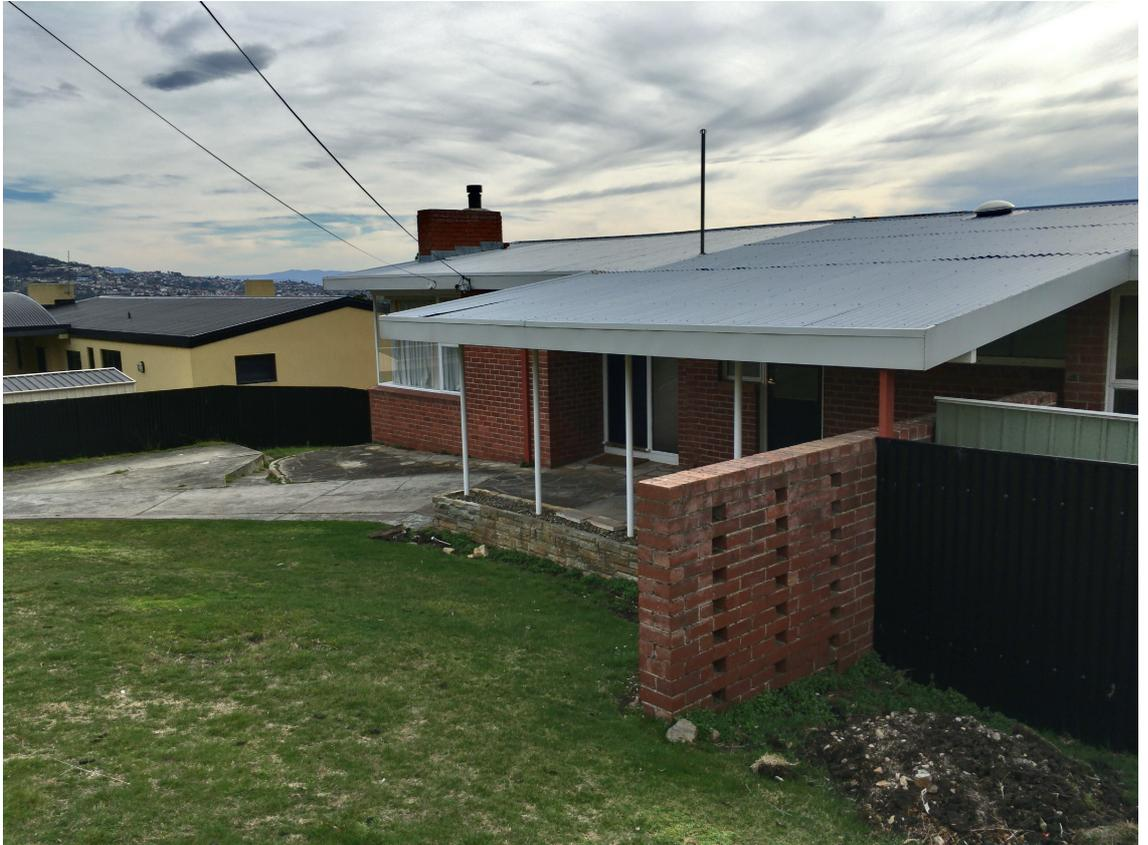
***Plate 3: The existing carport roof would be extended with a new skillion section for much of the length of the existing free-standing brick wall.***
