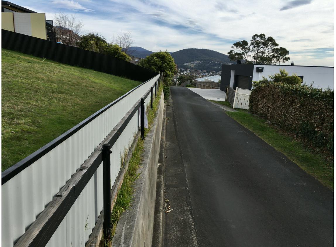
***Plate 4: The proposed rear access steps are to be cut into the existing concrete retaining wall on Niree Lane at the northern (rear) corner of the site and would for the most part be below ground level, cut into the sloping site.***
