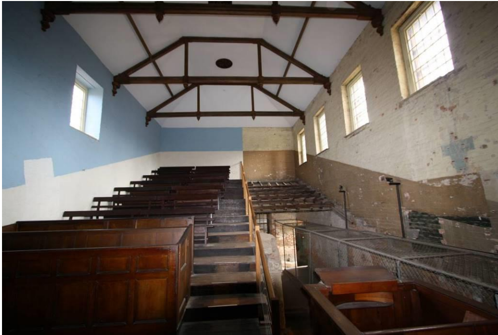
Plate 2: View south at the Chapel room showing the ceiling trusses where speakers 1-9 will be placed, and the areas where speakers 10-20 will be positioned, below seating or in voids
