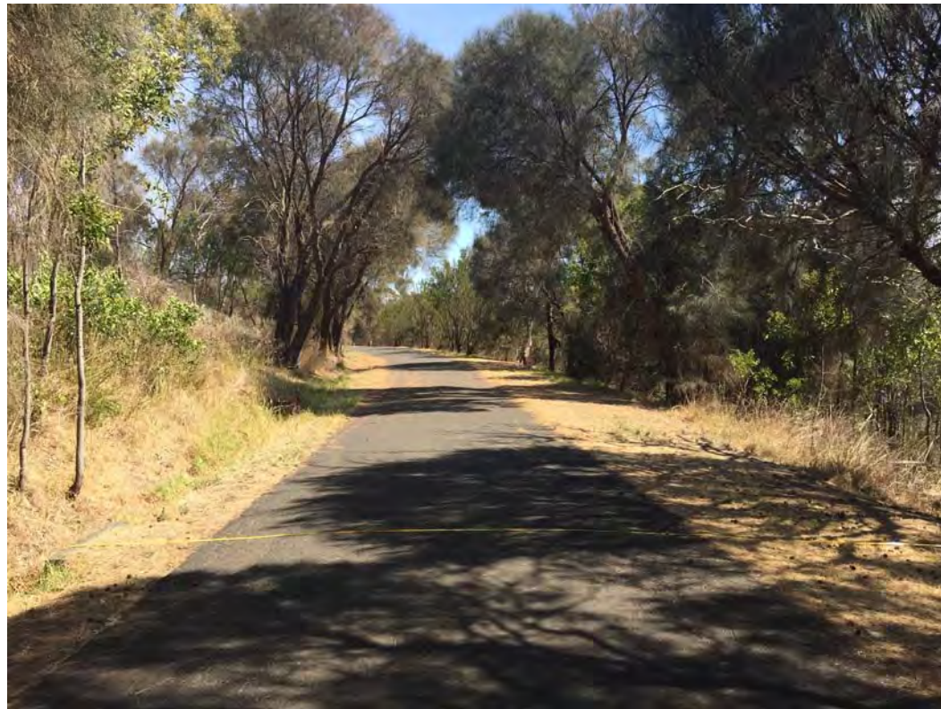
Existing conditions with drain on left, bitumen surface and edge of road (span of approximately 7.5m)
