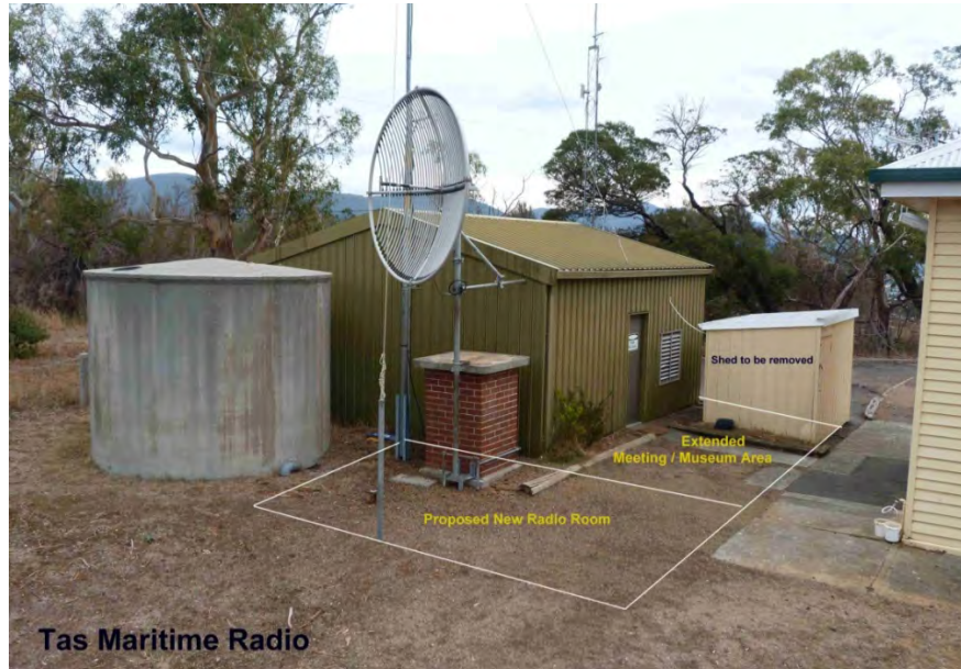
Photo 2. Approximate footprint of proposed shed extension.
