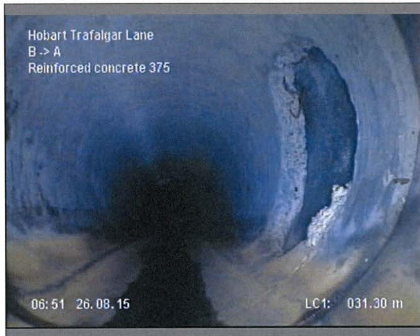
Photo: 1_15B, MPEG #: 260815_1, 00:12:52 31.3m, Point repair, hole repaired , length: 300mm , from 1 to 5 o'clock
