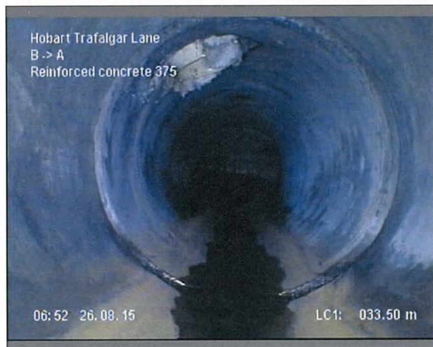
Photo: 1_17A, MPEG #: 260815_1, 00:13:40 33.5m, Joint displaced longitudinally, longitudinal displacement 21-30mm
