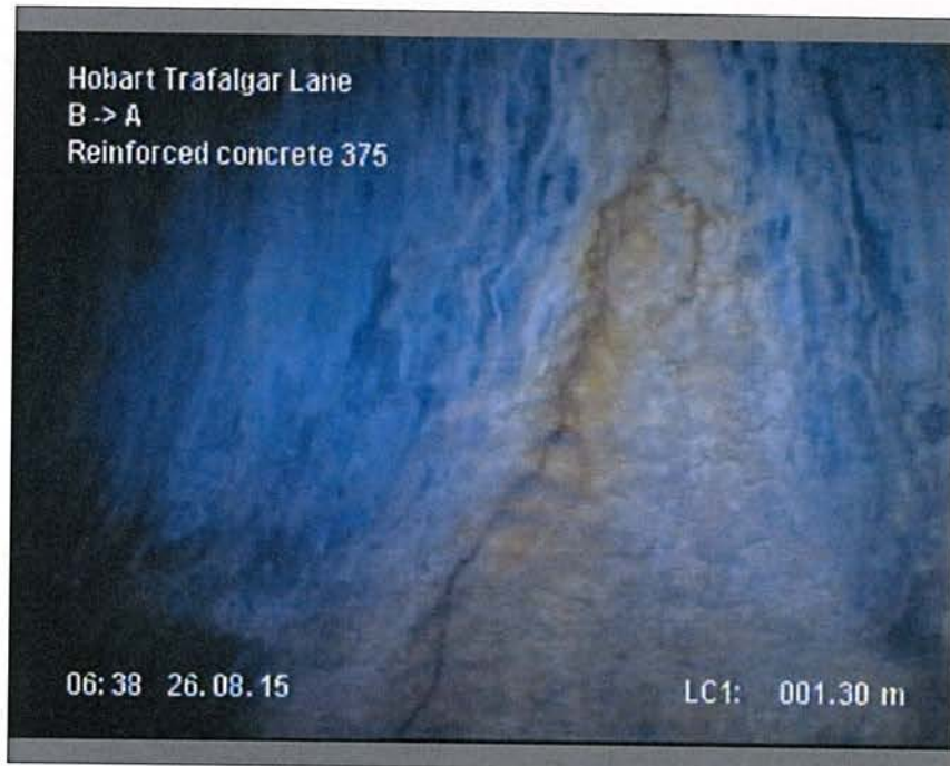
Photo: 1_2A, MPEG #: 260815_1, 00:02:45 1.3m, Circumferential fracture , width 3mm , from 12 to 12 o'clock
