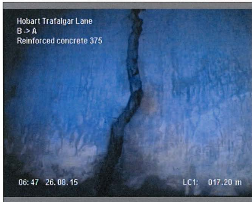
Photo: 1_9A, MPEG #: 260815_1, 00:08:58 17.2m, Circumferential fracture , width 5mm , from 12 to 12 o'clock
