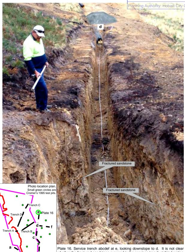
whether the fractured sandstone exposed in the services trench at this location (and locally elsewhere along it) is in-situ or not.
