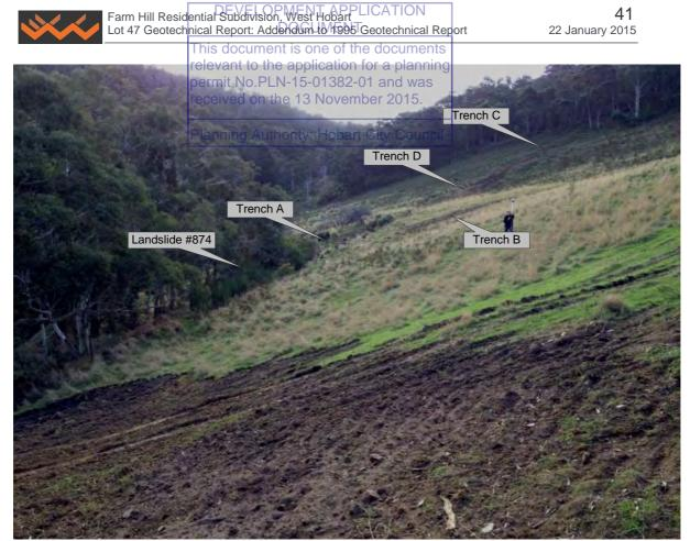
Plate 5 (above). View north over Lot 47 from its lower, southern boundary. The higher edge of the tree line in the left middle ground marks the headscarp of landslide #874 (see Map 1 of Attachment 5). Investigation trenches A,B, C and D are indicated.
