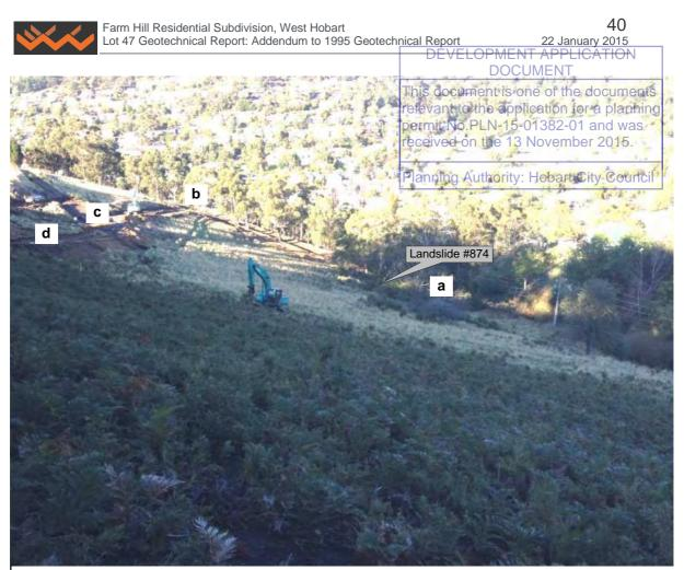
Plate 3 (above). View south southeast from the northwestern corner of Lot 47 at Farm Hill, over 25 – 300 slopes in the foreground, towards service trenches a....f (see Attachment 7). The higher edge of the tree line in the centre of the photo marks the headscarp of landslide #874 (see Map 1 of Attachment 5).
