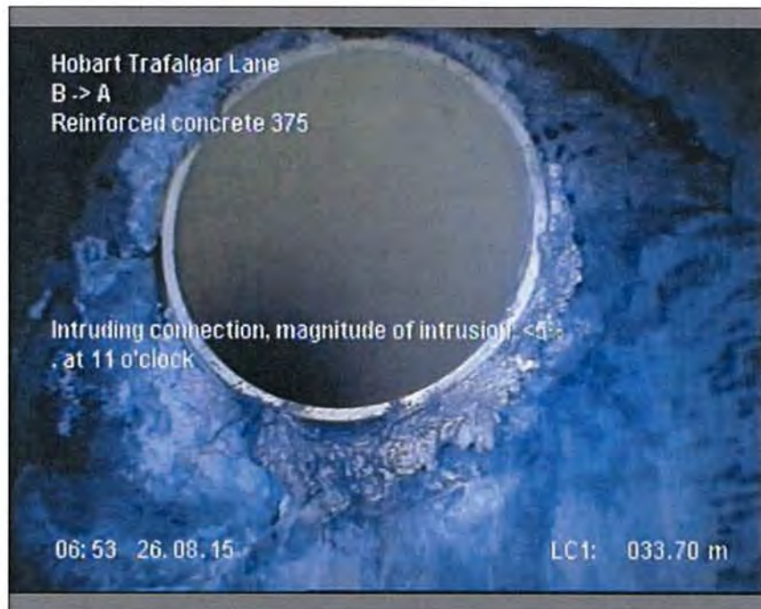
Photo: 1_19A, MPEG #: 260815_1, 00:14:07 33.7m, Intruding connection, magnitude of intrusion: <5% , at 11 o'clock
