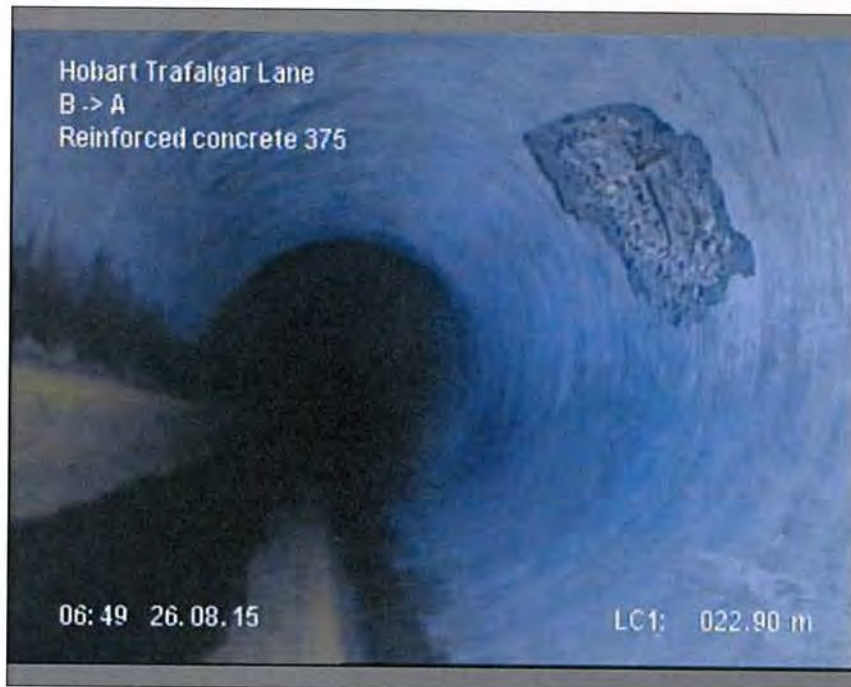
Photo: 1_11B, MPEG #: 260815_1, 00:10:27 22.9m, Spalling of the conduit fabric, localized chipping of one or more of each , Obstruction: <5% , from 12 to 2 o'clock
