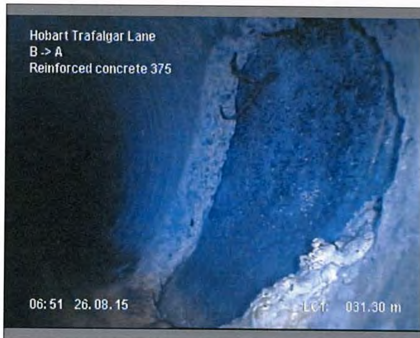
Photo: 1_15A, MPEG #: 260815_1, 00:12:52 31.3m, Point repair, hole repaired , length: 300mm , from 1 to 5 o'clock
