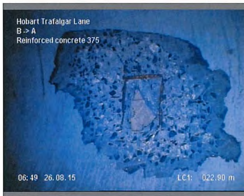
Photo: 1_11A, MPEG #: 260815_1, 00:10:27 22.9m, Spalling of the conduit fabric, localized chipping of one or more of each , Obstruction: <5% , from 12 to 2 o'clock
