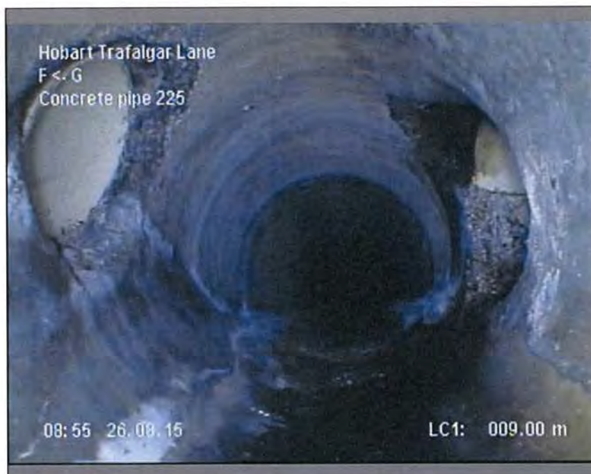
Photo: 6_5B, MPEG #: 260815_1, 00:12:54 9m, Connection, good workmanship, connection appears to be open, height 100mm , at 2 o'clock, PVC
