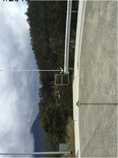
600 VEE DRAIN INSTALLED AROUND PERIMETER OF CUL-DE-SAC
