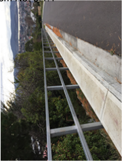
EXAMPLE OF PROPOSED VEHICLE BARRIER TO REPLACE SHORT SECTION OF GUARD RAIL BETWEEN U1 AND U2 DRIVEWAYS. VEHICLE BARRIER TO EXTEND THE LENGTH OF BOTH U1 AND U2 DRIVEWAYS
