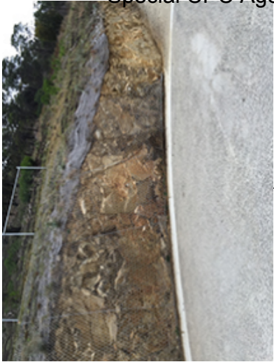
600 VEE DRAIN INSTALLED AROUND PERIMETER OF CUL-DE-SAC
